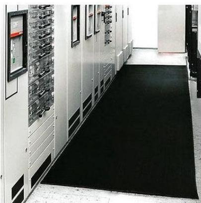
SAIVI Electrical Insulating Mats 10KV to 50KV.
